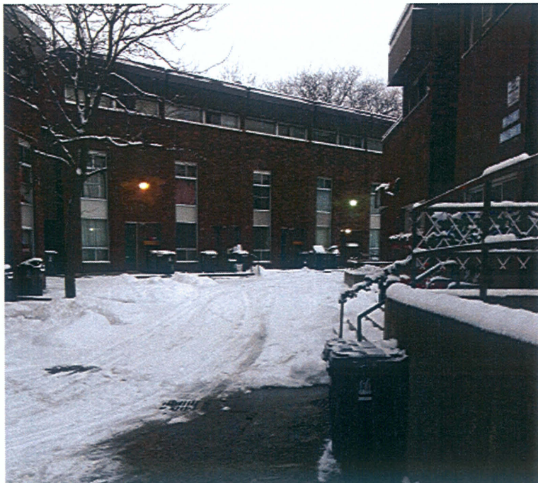
Photograph 5: View of townhouse units along Vanaulay Square, looking east. ALEXANDRA PARK – 35 to 56 VANAULEY COURT and 57 to 74 VANAULEY SQUARE TORONTO, ONTARIO
