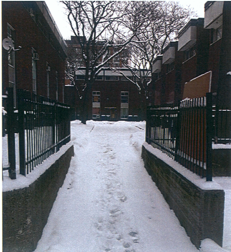
Photograph 2: View of townhouse units on Vanauley Court, looking east.
