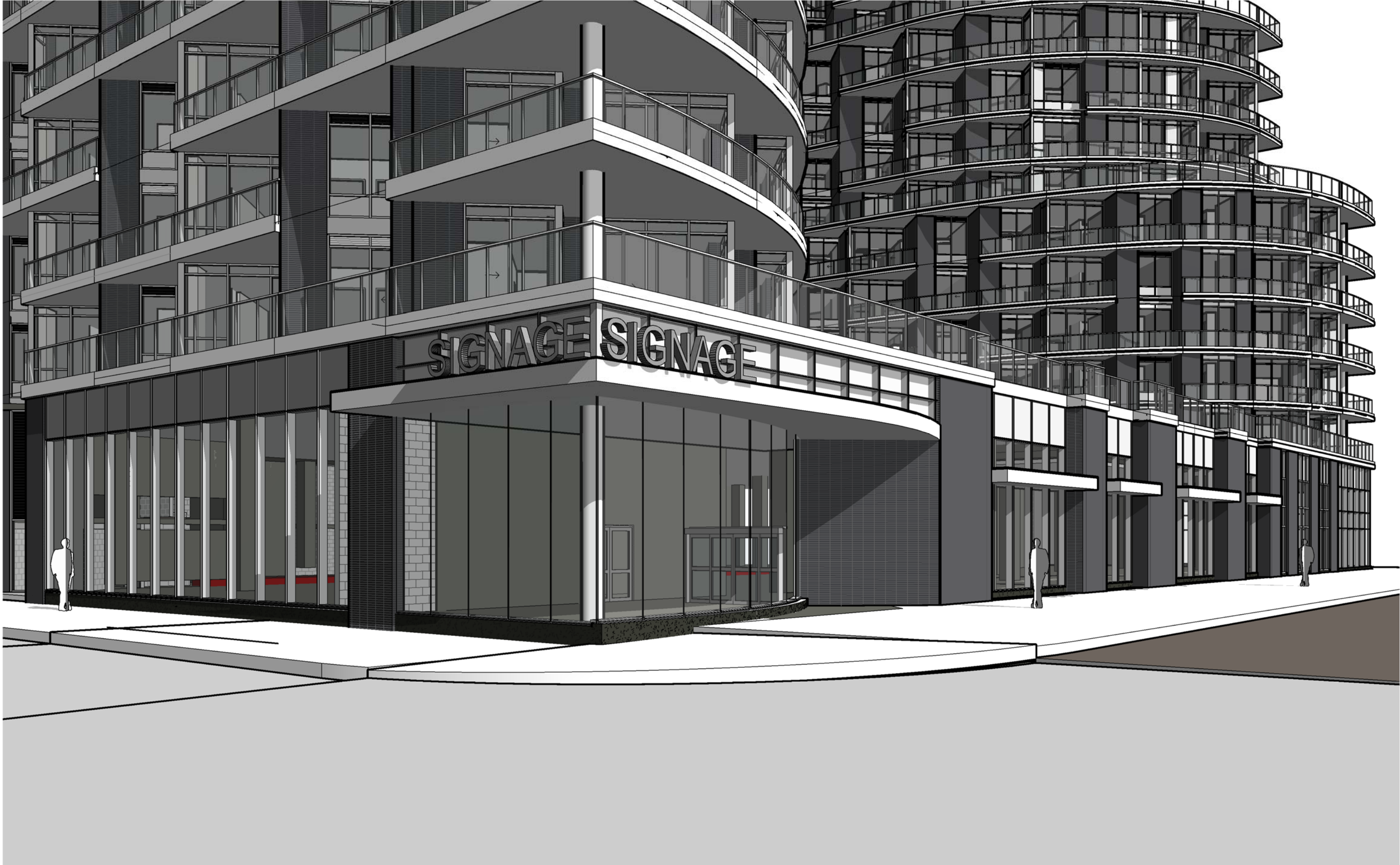
OPTION E - curved entrance SW corner only + recessed glass storefront with canopies + brick piers
